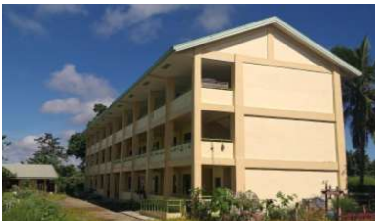
Figure 2. Three Storey SHS Building of Trento National High School
